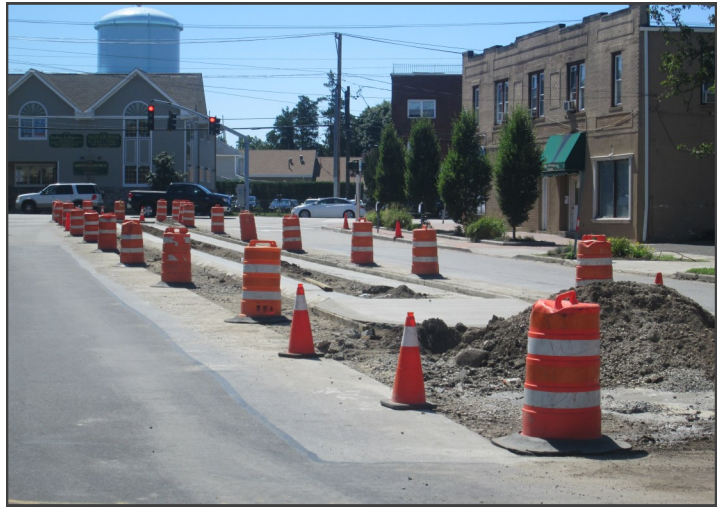
A center lane median is being constructed on Hillside Blvd. Plantings will be done in the Fall.
